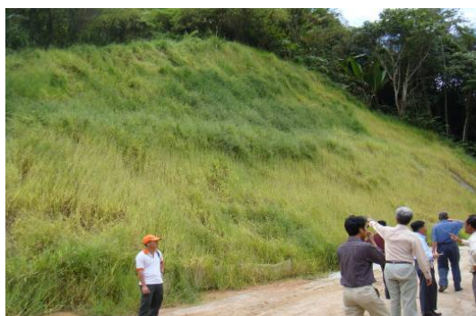
b) Completed Hydroseeding
