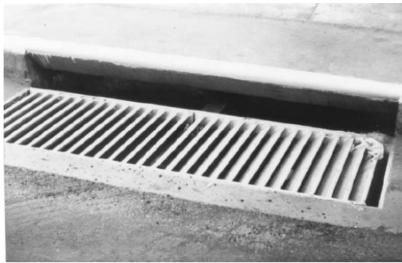
Figure 13.5: Combination Curb-opening, 45 Degree Tilt-bar Grate Inlet
