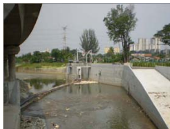
a) Floating Debris Trap - Type 1
