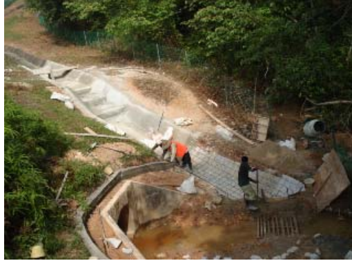
Figure AX2.10: Maintenance Work for Culvert
