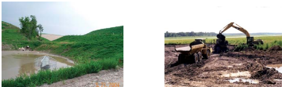
Figure AX2.6: Sediment Removal Work
