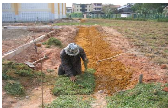
a) Turfing in Progress
