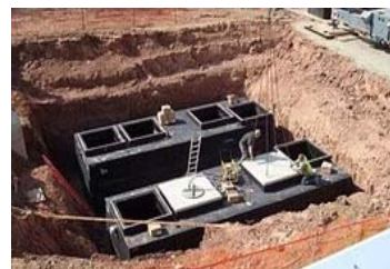
d) Oil and Grease Interceptor - Type 3
